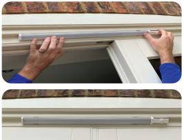
Screw the 2 mounting clips about 40cm apart to the wall (or overhang) with the supplied screws. The distance between the clips isn't critical as they can fit on anywhere along the length of the aluminium part of the light.
